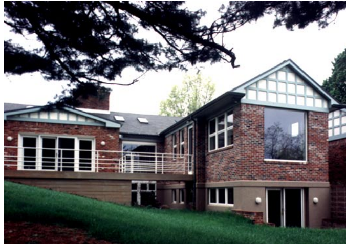
finished rear view
