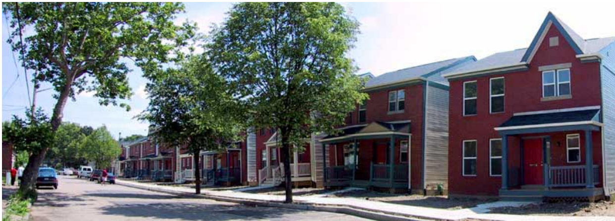
MELLON STREET UNDER CONSTRUCTION
