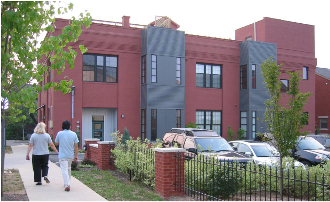
View after renovation
